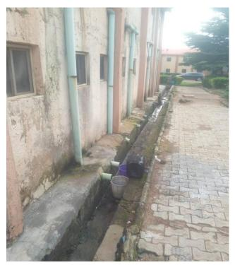
**Figure 1**. Grey water collection from drainage pipes in Adeniyi hostel, FUTA.
