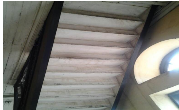
Figure15: Wooden part of the staircase
